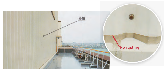
Outer walls of Okinawa Thermal Power Station (Coastal, 27 years after installation)
